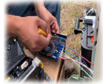
Fiber Optic Cable Splicing
